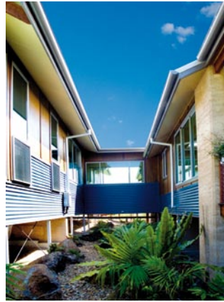
Rammed earth house, Currumbin.
