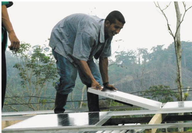
Members of the San Jose de Apartado village fit solar panels.
