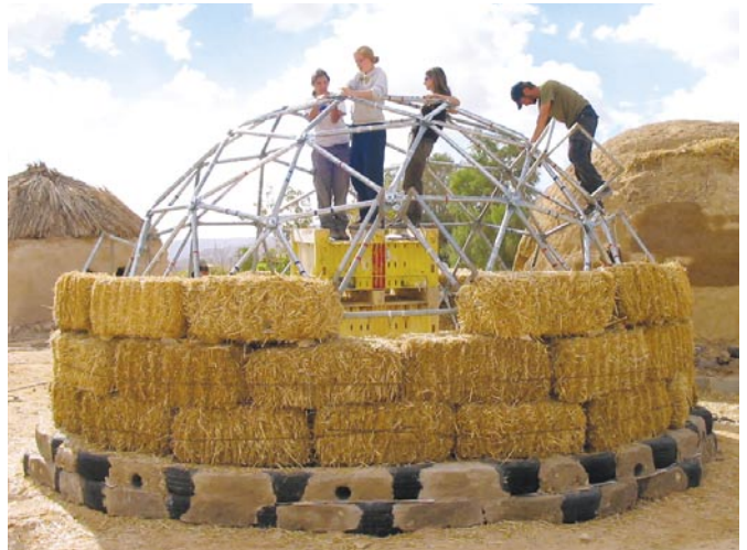
Construction of a strawbale building at Arava Valley, Israel.
