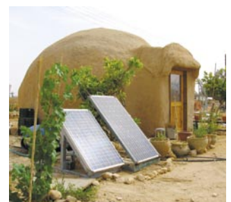
A completed building with solar panels.
