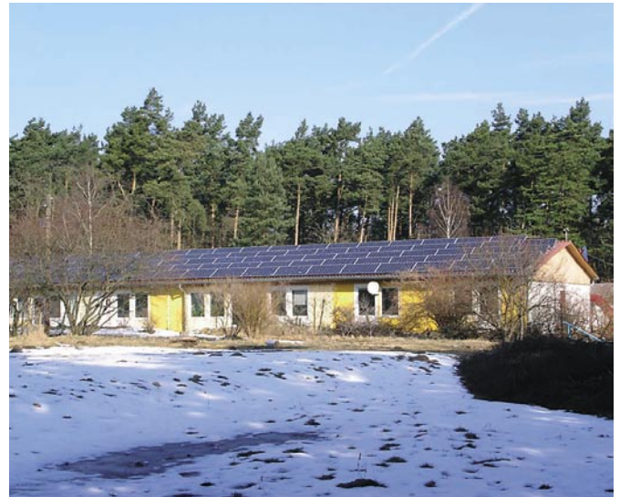
Photovoltaic panels on one of the buildings at ZEGG.
