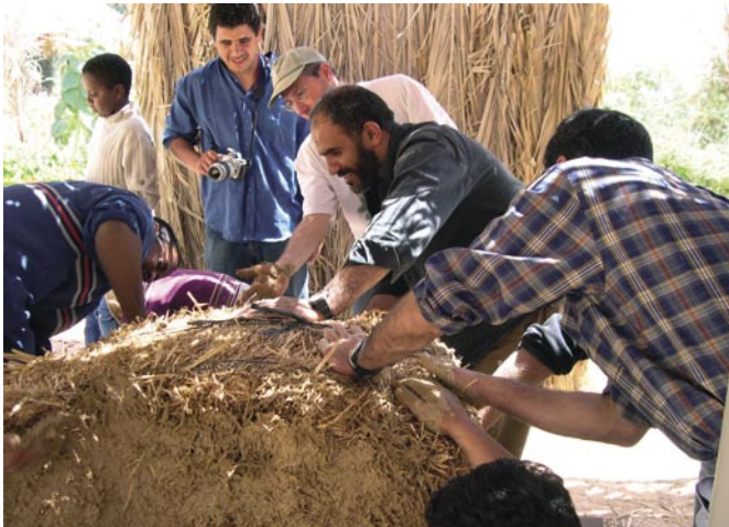
Ecological building work underway at Kibbutz Lotan, Israel.
