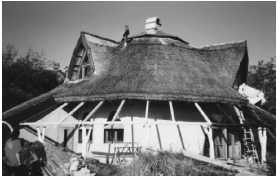
Straw roof on a compressed earth house at Gyurufu, Hungary
