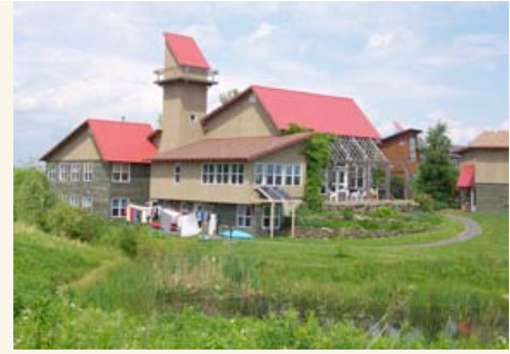
FROG's Common House includes large triple-glazed, passive solar windows on the south side and laundry hung out to dry on the clothesline.
