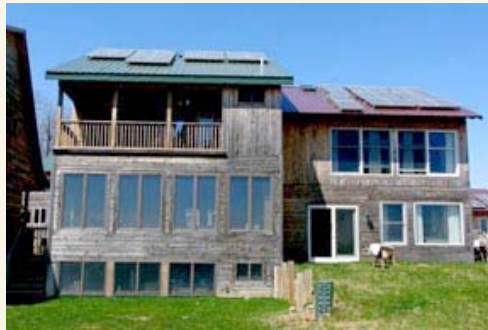
Almost half of SONG homes have photovoltaics on the roofs and generate electricity from the sun.
